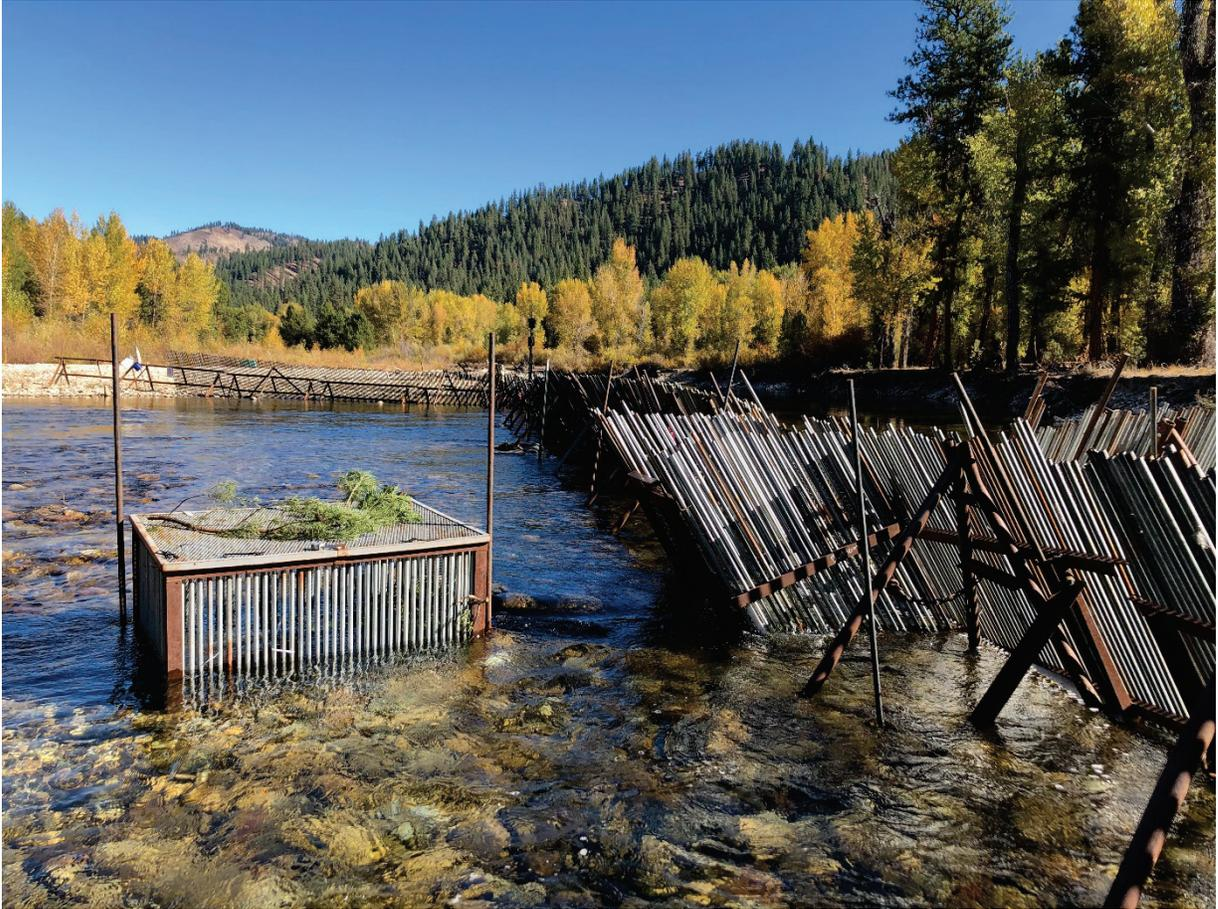
**Figure 7. Downstream trap box. The V and rectangle created by pickets is similar to the upstream box with an additional tube connection for fish to move downstream into the trap box. Photo credit: Mark Nelson.**
