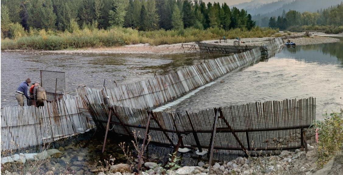
**Figure 4. Photo of the North Fork Boise weir (2021). Flow is from right to left. Staff is standing at the open downstream trap box. Photo credit: Jaan Kolts.**
