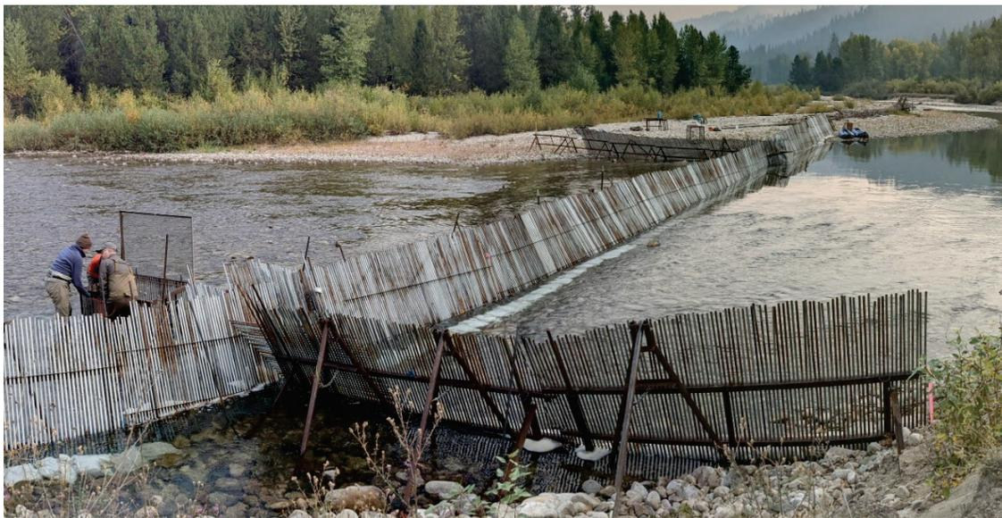
**Figure 12. Photo of the North Fork Boise River weir (2021). Flow is from right to left. Staff is standing at the open downstream trap box. Photo credit: Jaan Kolts.**
